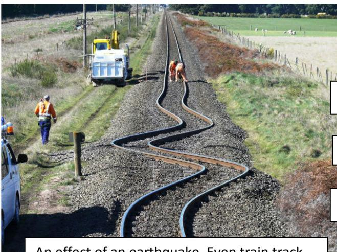
An effect of an earthquake. Even train track can change as and effect of an earthquakes.
